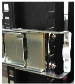
3. Repeat Step 1 and 2 for another slide-rail assembly in order to install in onto the rack.
